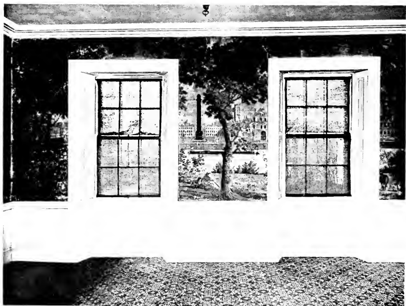
PLATE LXXXIII.—Wall of Parlor, Cook-Oliver House, showing “Panorama of Paris” Wall Paper; Embrasured Windows with Folding Shutters.
